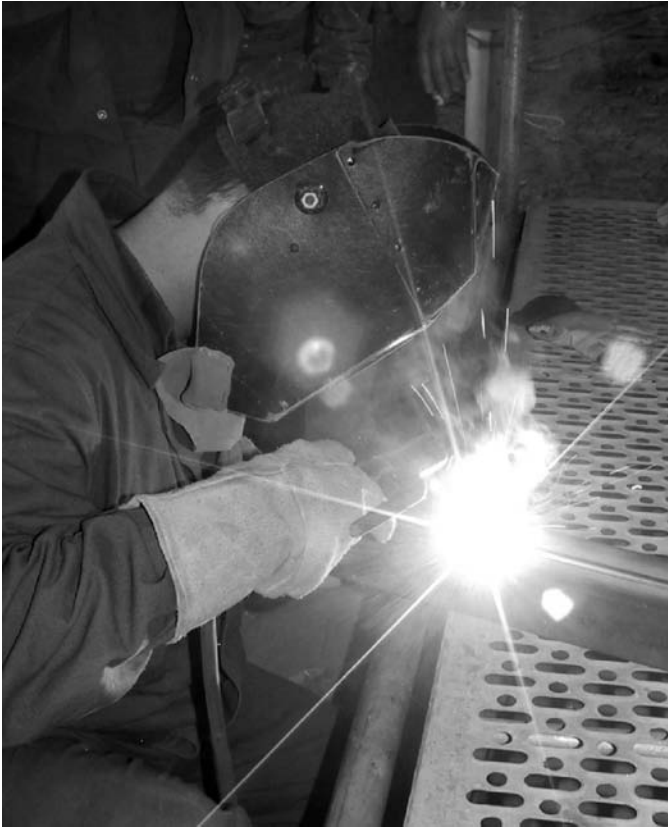
FIGURE 13.4 Electric arc welding.
