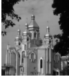
Church of St. Andrew in Drohobych
