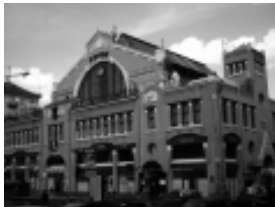
Bessarab Market in Kyiv by architect Henryk Gaj (1910)
