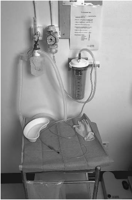
Fig. 1: Wall suction unit and oxygen delivery system.
